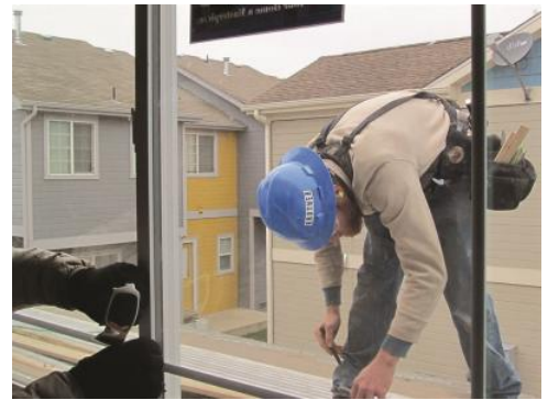
A volunteer works just outside a second-story bedroom window.
