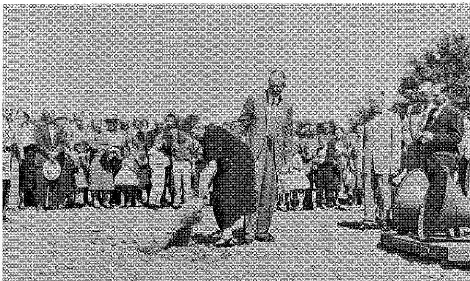
Ground-breaking at 350 Eleventh Avenue
